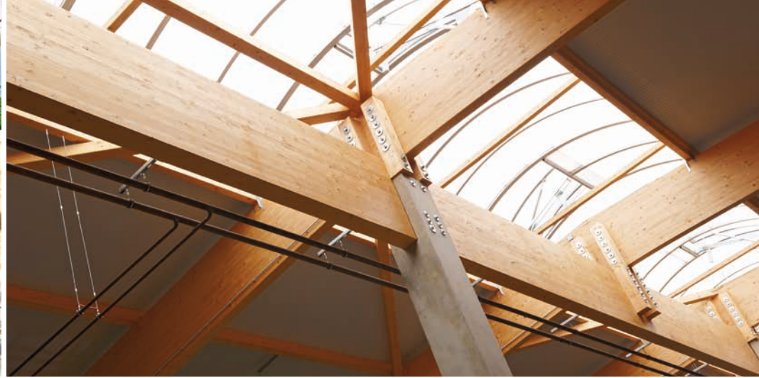
Built by Holzbau Kühlborn based in Spangenberg, Germany
