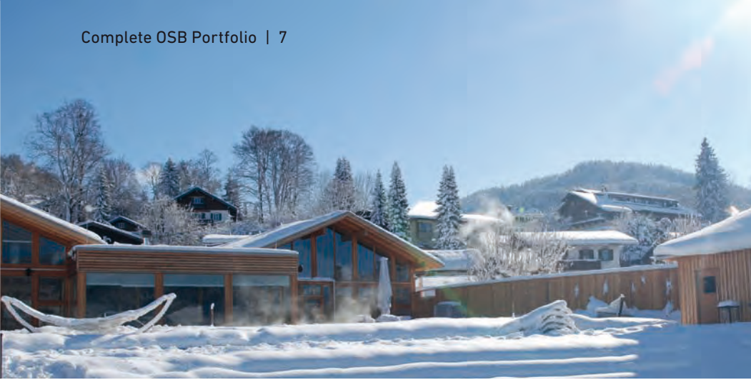
Monte Mare Sauna at Lake Tegernsee, Germany
