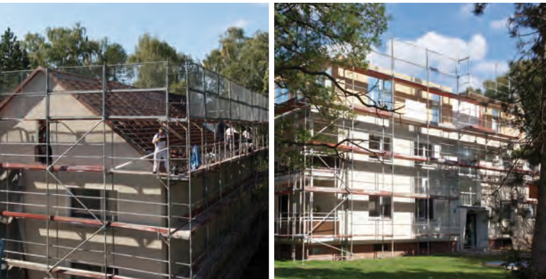
Built by Opitz Holzbau based in Neuruppin, Germany
