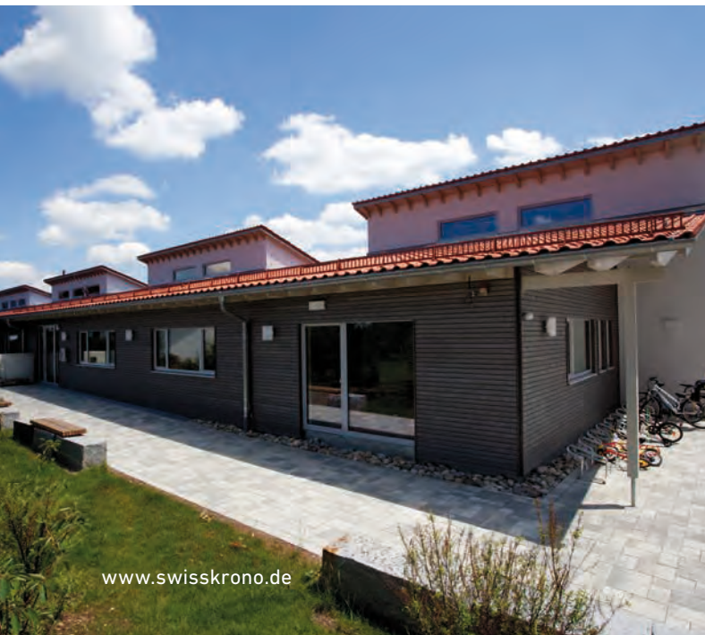
Built by Hubert Schmid Bauunternehmen based in Marktobendorf, Germany
