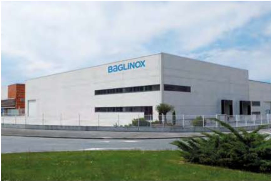
Fábrica / Factory / Usine. Orcoyen, Navarra
