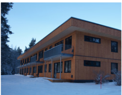
binderholz Lakehouse apartment block, Lieksa | Finland
