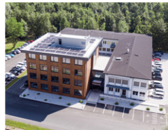
binderholz TimberBrain Office Building, Hallein | Austria
