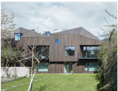
Private semi-detached house Mut zur Lücke, Innsbruck | Austria
